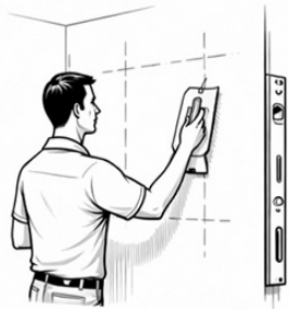
1. Prepare Wall and Apply Adhesive
