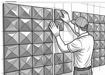
3. Press and install the tiles
