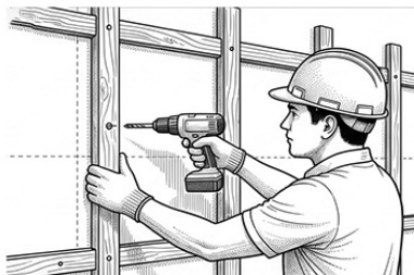
2. Install Wooden Furring Strips
