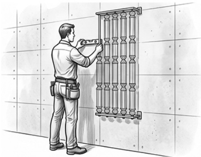
3. Interlock and Level Remaining Panels with Integrated Tabs
